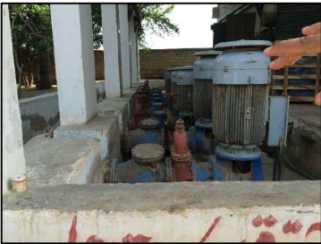
5+4 Vertical Turbine Pumps 3 Pumps of 100HP 2 Pumps of 220HP
