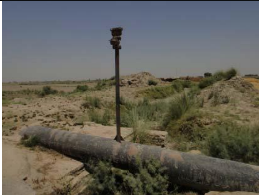
PICTURE-5: EXISTING RISING MAIN: Air valves of this rising main will be repaired and / or replaced
