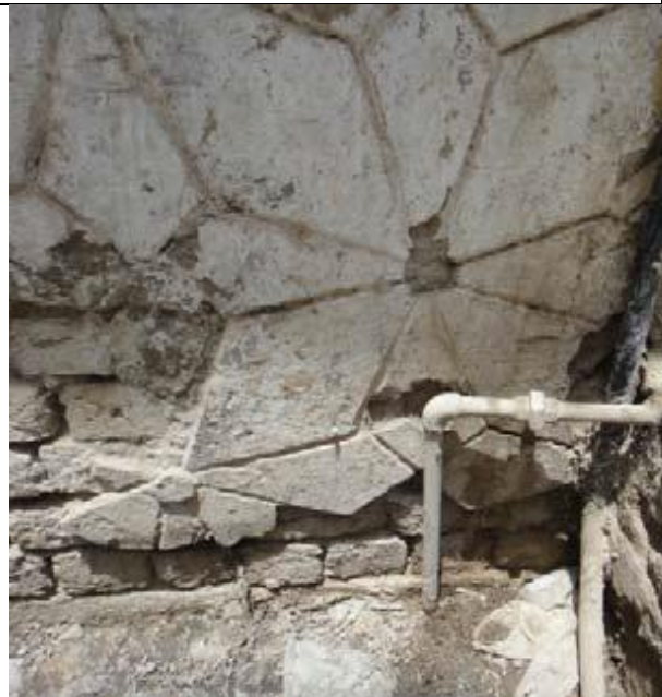
PICTURE-6: EXISTING WATER CONNECTIONS TO HOUSES: Their dilapidated conditions result into many water losses and contamination issues.
