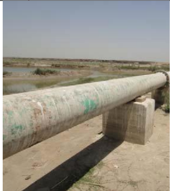
PICTURE-2: VIEW OF GRAVITY PIPE TO EXISTING RAW WATER POOLS: A similar pipe will be laid for the proposed pool # 3
