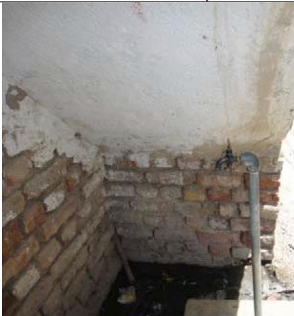
PICTURE-6: EXISTING WATER CONNECTIONS TO HOUSES: Their dilapidated conditions result into many water losses and contamination issues.
