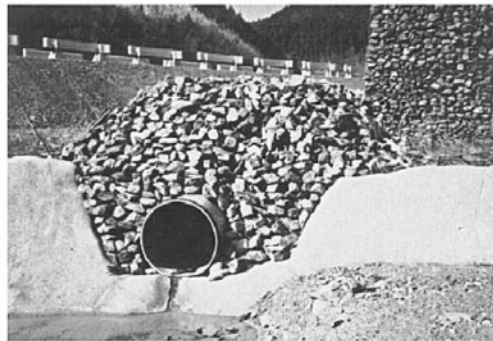
Picture2-13 Example of bottom leachate collection pipe and gas venting pipe
