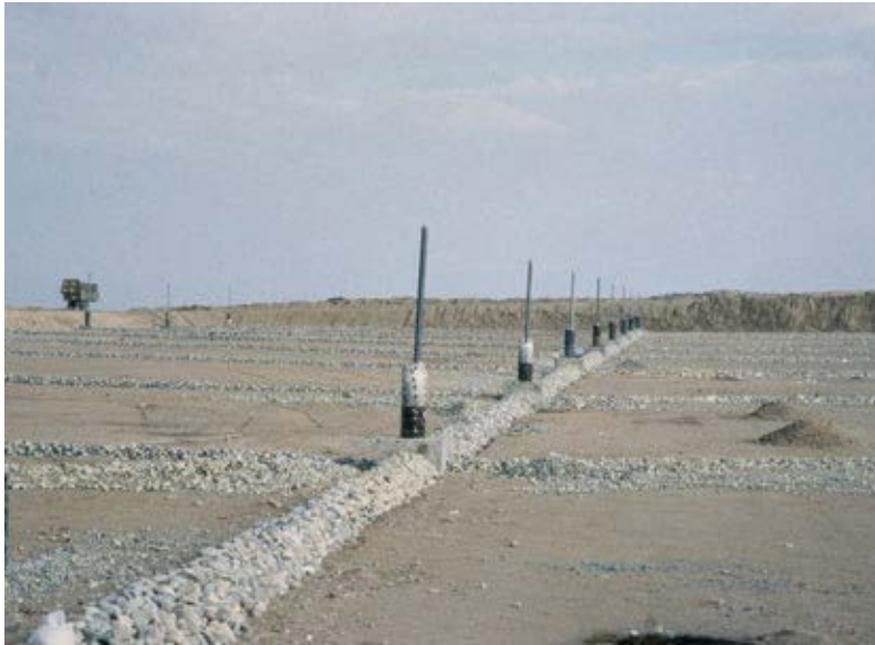
Picture 2-10 Installation example of gas venting pipes
