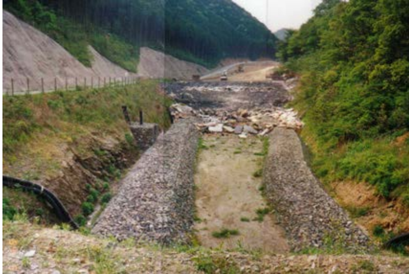
Picture 3-3 Example of landfill of rough waste material in the vicinity of leachate collection discharge pipe
