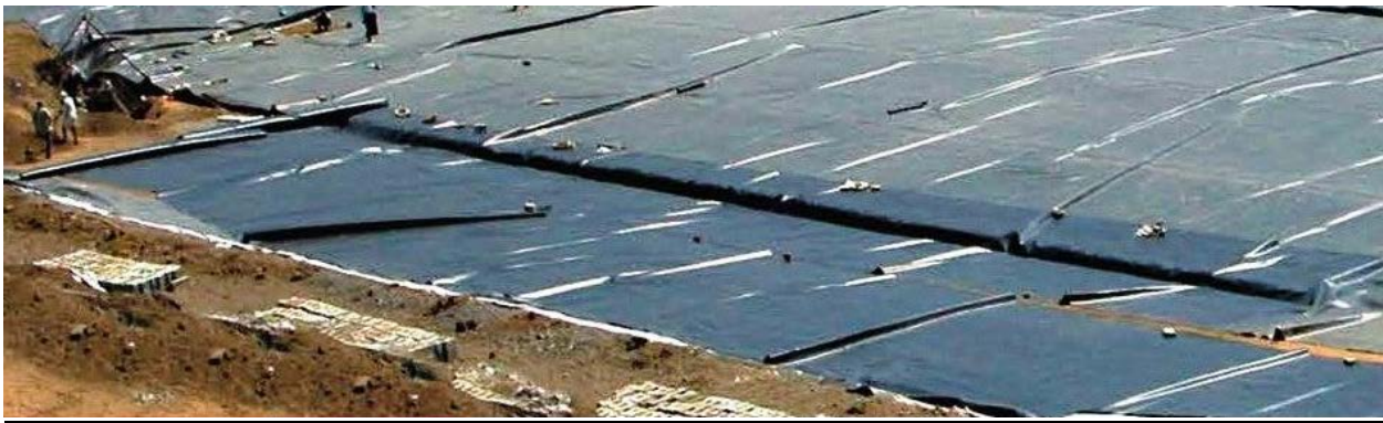
LINING ARRANGEMENTS OF GEO MEMBRANE
