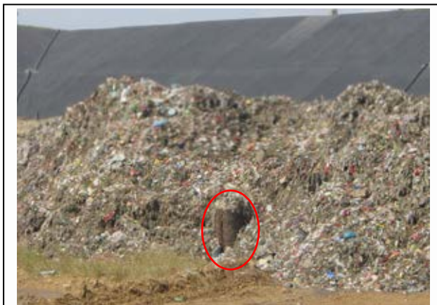
Picture 3-8 Waste is higher than Gas venting facility (○) case (bad example)
