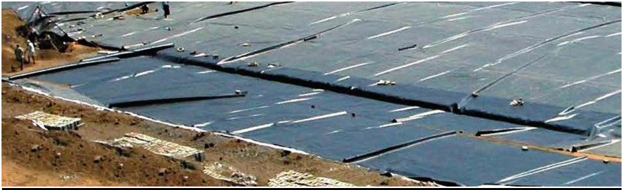
LINING ARRANGEMENTS OF GEO MEMBRANE
